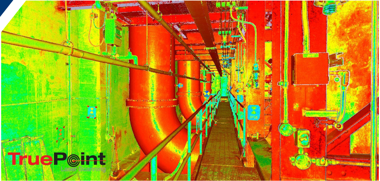
TruePoint provided 3D laser scanning for a sewerage pumping station, capturing all structure, MEP and piping down to ½" diameter.
